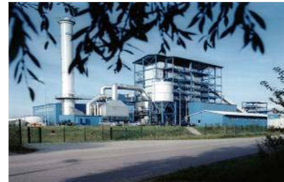
Modern Co-generation plant
