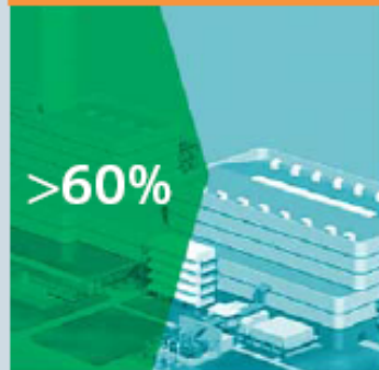
Irsching 4 plant 530 Mw
